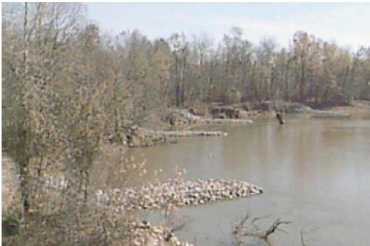
Figure 16: Photograph of bendway weirs. USDA NRCS 2013.
